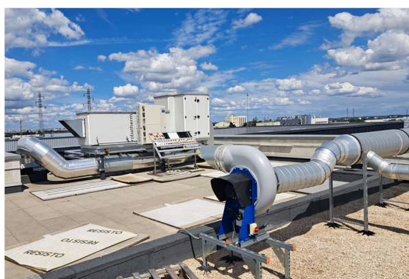
Figure 35 Air extraction and fresh air compensation system (CTA) on the roof for efficient air extraction on the laboratory
