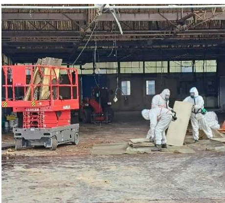
Figure 37 Dismantlement of the asbestos-containing buildings #3/#6 and #12 (left picture), new implemented solvent extraction system (middle picture), new IBC at the mixing station (right picture)
