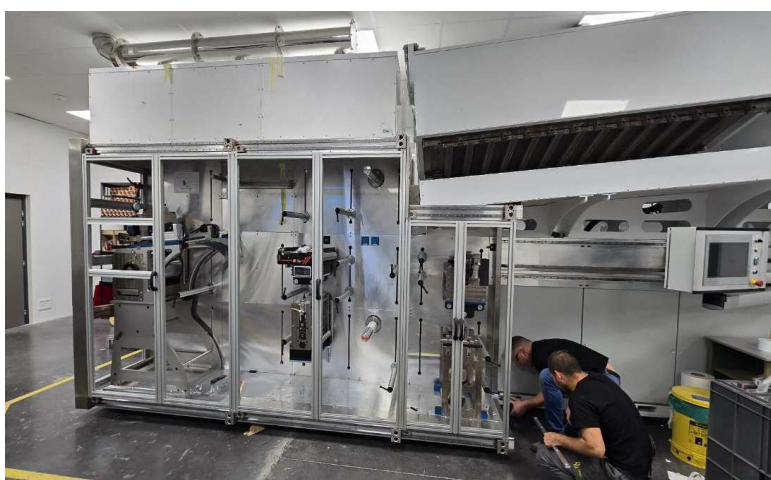
Figure 36 Confined Adhex industrial pilot line (2024-2025): coating tunnel confinement absorbing the VOC and treating ozone, installation of an improved human-machine interface and additional measurements systems (like explosion limit detector)
